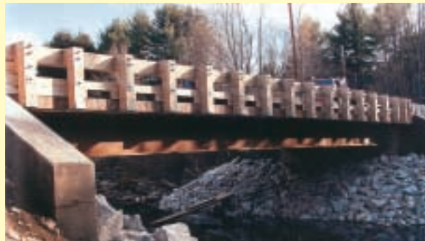
SKIDMORE BRIDGE UNION, MAINE
