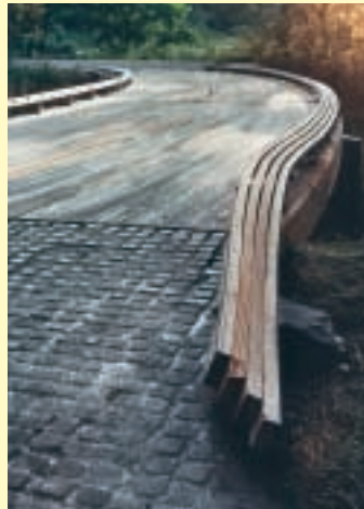
IL POGGIO BRIDGE WASHINGTON, CONNECTICUT
